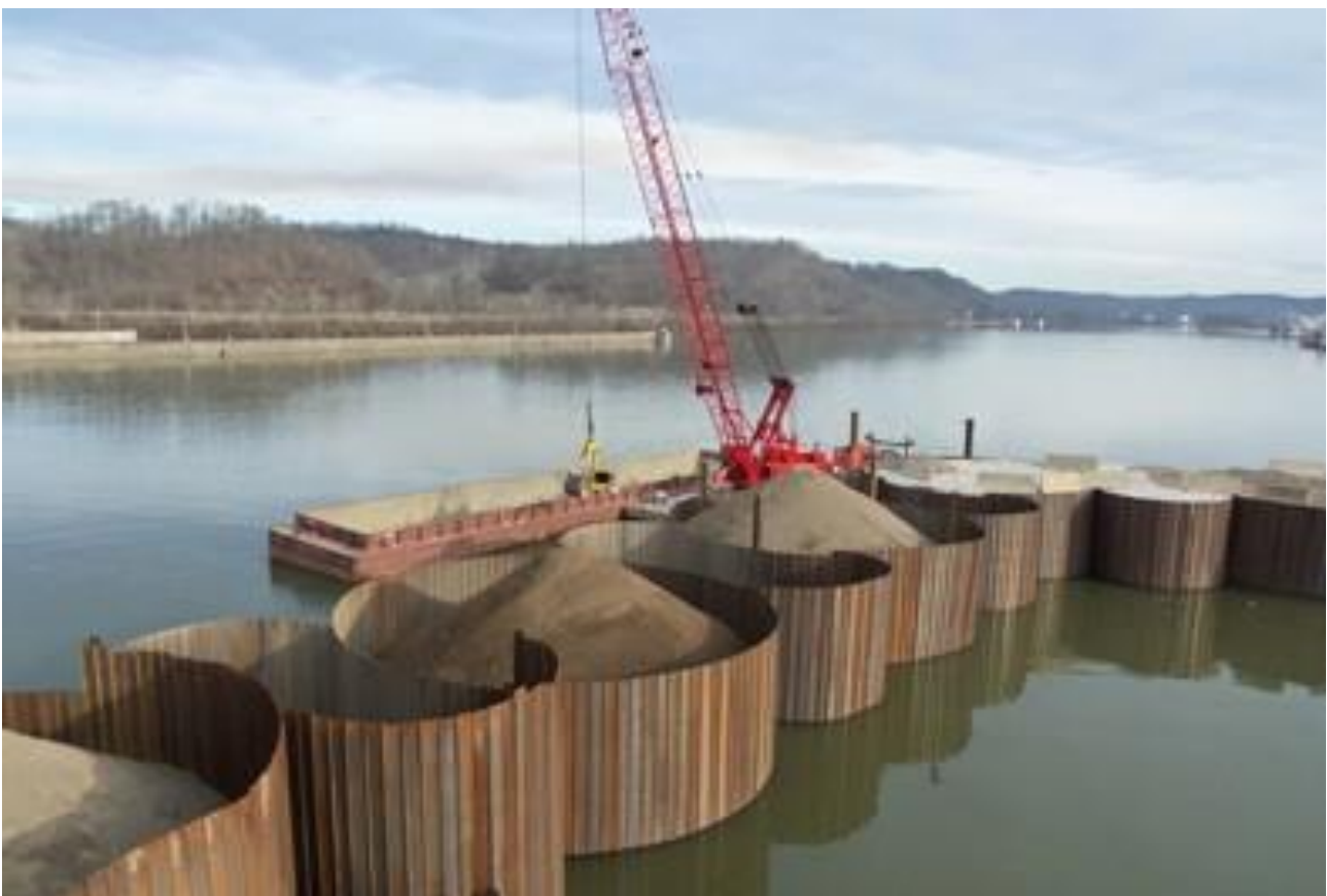
Figura 8. Cofferdams o Ataguías. Photo of Cellular Cofferdam. Photo from C.J. Mahan Construction Company.
