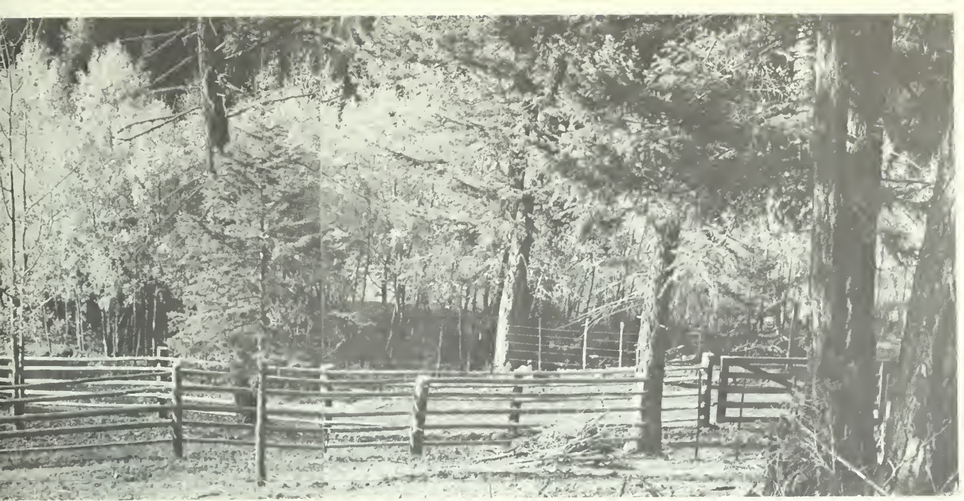
Cattle handling facilities at Pass Lake
