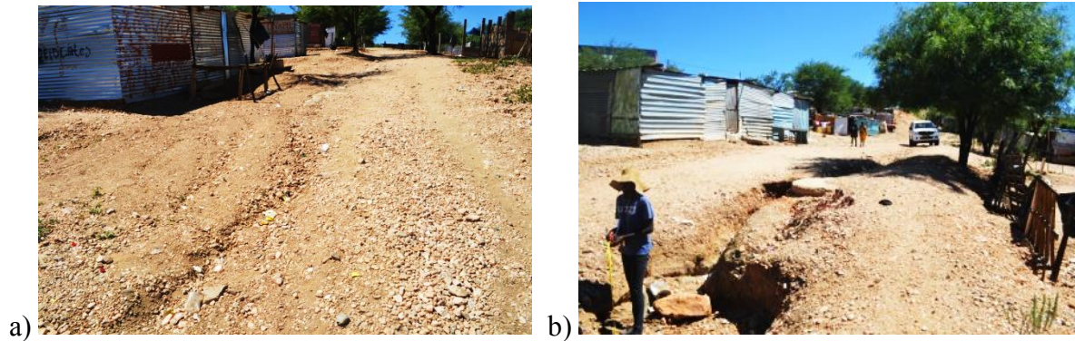
Figure 1: Photographs on: a) Rills, b) Gullies with damages to road. Source: Shikangalah RN.
