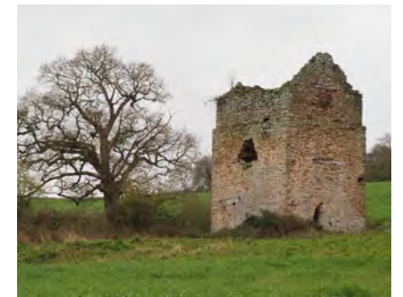
2. Copper mine engine house, Dodington
