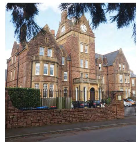
2. Former hospital administration block
