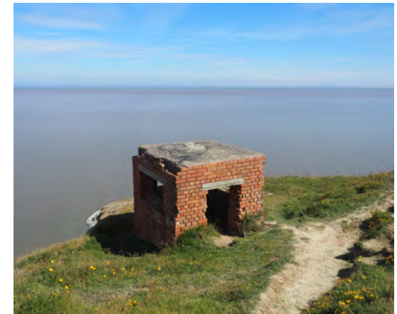
2. WWII look out on cliff top, with views across the Bristol Channel
