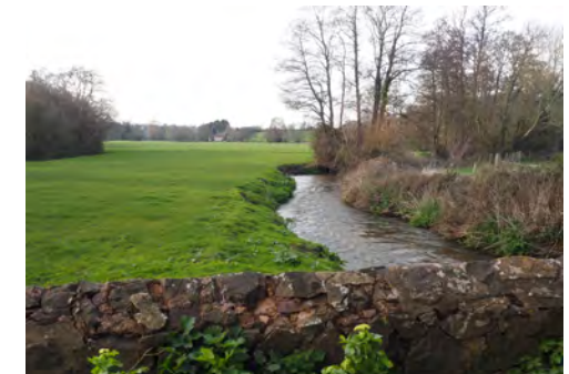
2. Historic bridge over the Doniford Stream near Cottiford
