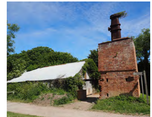
5. Oil Retort at Kilve (Listed Building)
