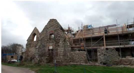
1. Kilve Chantry under repair
