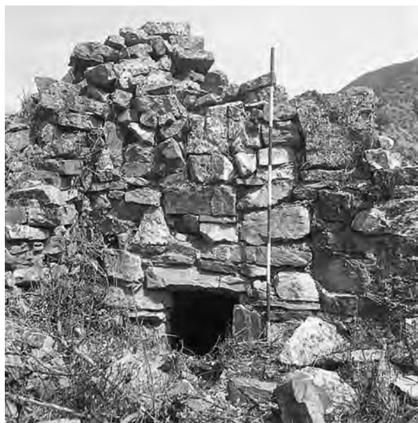
Fig. 11. Cayash Ragaj. Entrance to the burial chamber in the terrace wall. Photo: K. Tunia.
