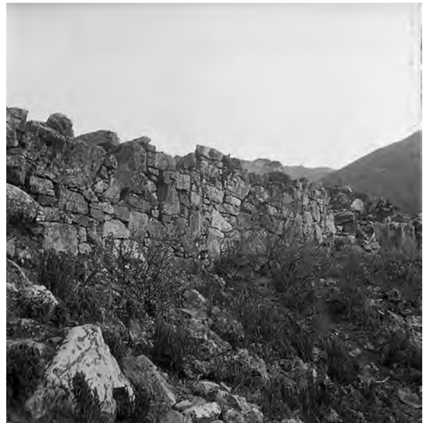
Fig. 9. Cayash Ragaj. The wall surrounding the settlement. Photo: K. Tunia.
