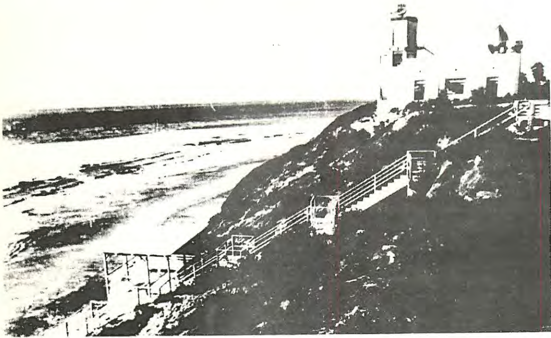
Figure 3A. Looking Northwest at the Self Realization Temple in Encinitas, California. The Temple was one of four buildings along these cliffs in 1939, was 4 stories high, and appeared to have an adequate bluff-top setback at that time. Photo: Self Realization Fellowship, Encinitas, 1939.
