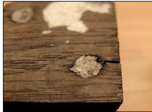
Fig. 4.31: Detail of the two holes filled with a low melting lead-tin alloy.
