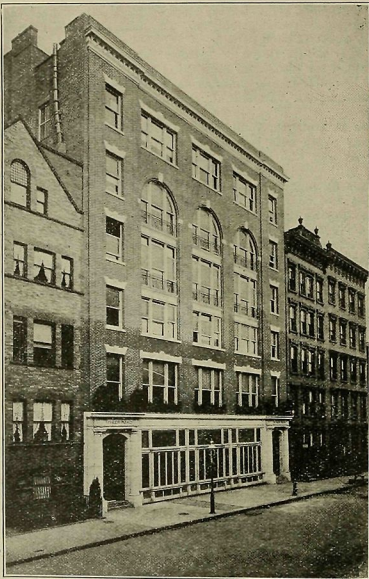
DOUBLEDAY, PAGE & CO.'S NEW BUILDING.
