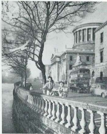
AR LAN LIFFEY—Y "FOUR COURTS"
