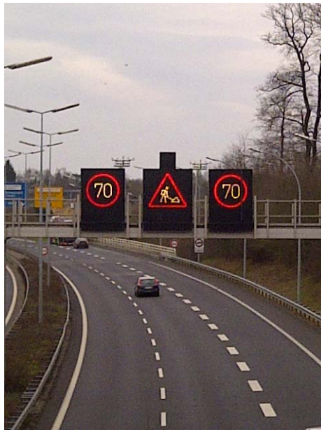
Figure 51 : exemple de panneau à message variable (Source : By GilPe [CC BY-SA 3.0] ( https://creativecommons.org/licenses/by-sa/3.0/ ), from Wikimedia Commons)
