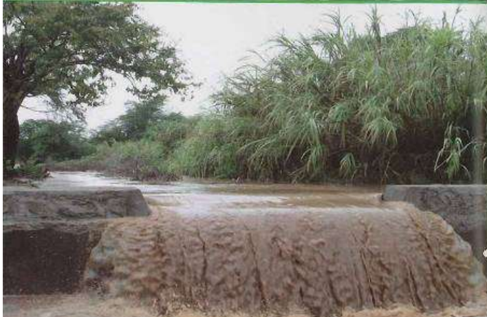
▲ Sand dam in dry season in Kitui district, Kenya (photo: Barst & Haas). Sand dam overflowing in wet season in Kitui district, Kenya (photo: M. Hoogmoed).
