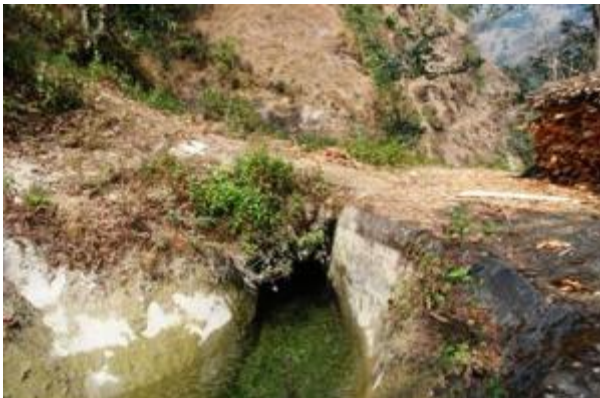
Tunnel of Small Hydropower project, Barnalu-1,
