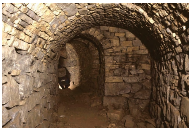
Figure 1. Stone arching in the Handsome Mea Flats near the area now called the 'Wheel Flats'. The image shows an area used to store ore trucks.
