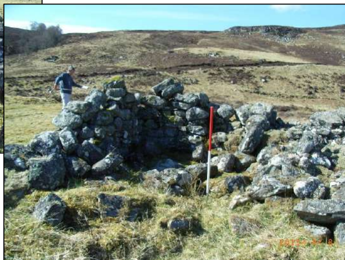
Figure 229: Building B151 – interior NW gable, looking NW
