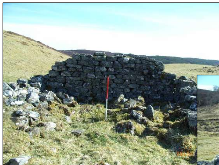
Figure 228: Building B151: interior of SE gable, looking SE
