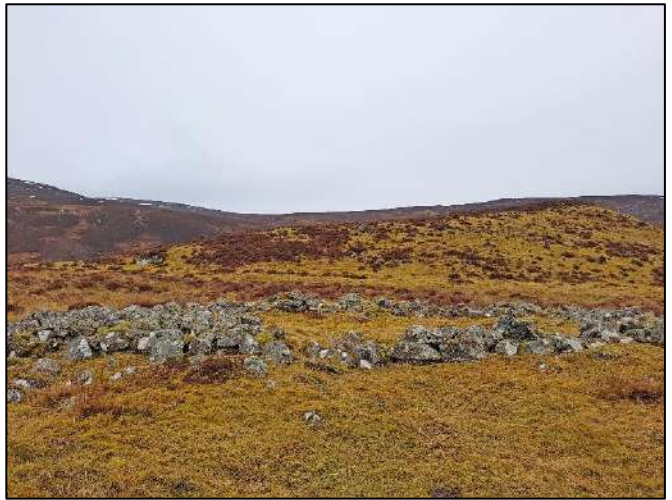
Figure 190: Building B103, looking SW
