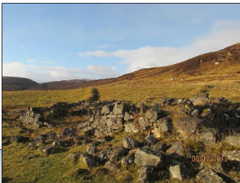
Figure 160: Photo taken from the eastern part of building, B104, along the line of the building. Looking W.
