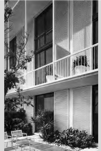
Palm Beach Apartment Complex
