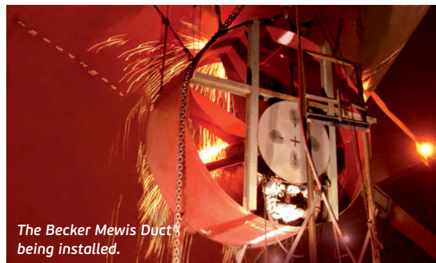
The Becker Mewis Duct® installed on the Bow Flora.
