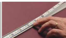
Lay Light In Channel
