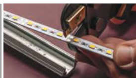
Measure & Cut Thin Strip Where Marked
