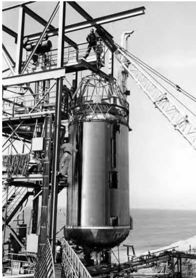
Figure 1: Image of the liquid hydrogen fueled Centaur upper stage during construction. (1)
