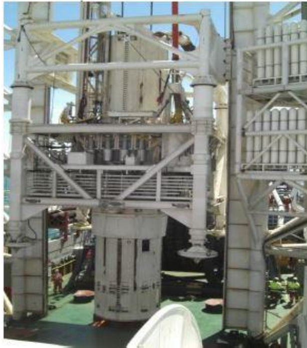
Figure 3: The 2.5 m diameter drill bit within the drill frame structure.
