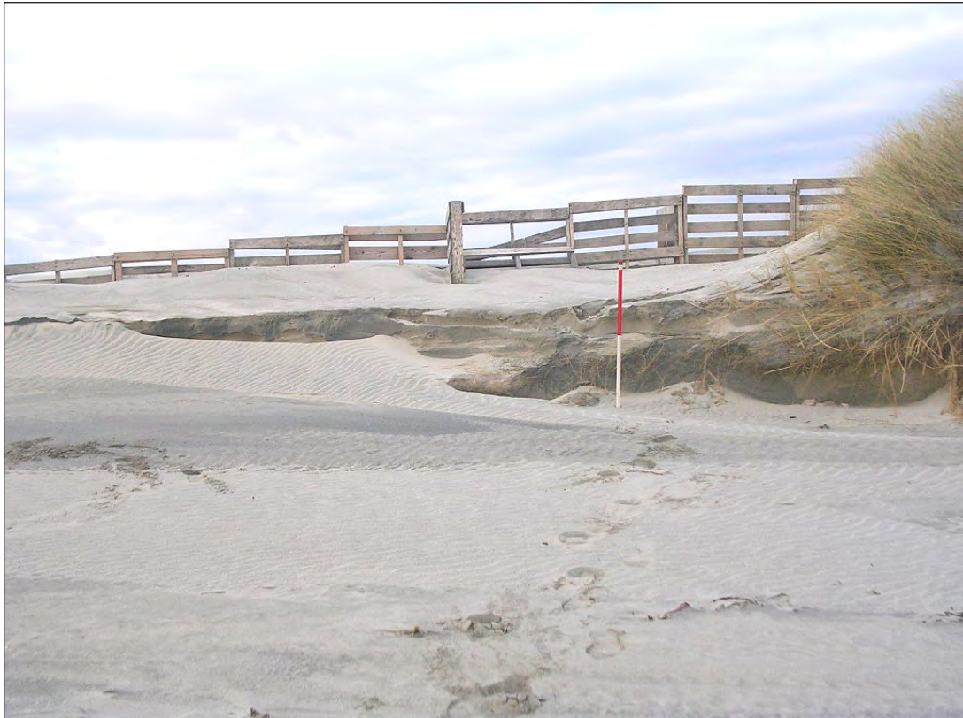
Plate 3 - Attempts to prevent or slow erosion using pallets, Tràigh Ear ( Coastal Geomorphology Cell 27 ).
