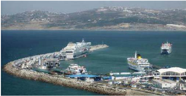
Port of Tanger Breakwater from W
