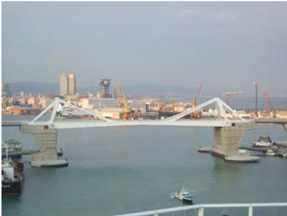
Barcelona—Bascule bridge at N end of Darsena del Morrot
