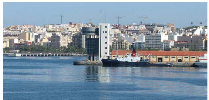
Ceuta Harbor Control Tower
