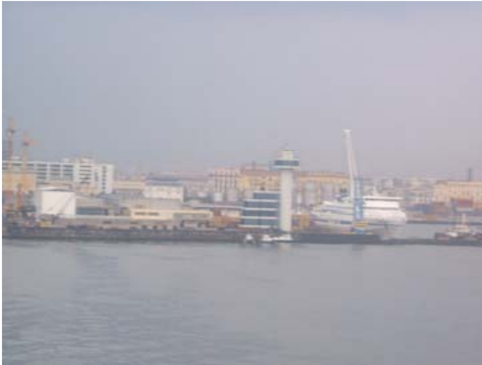
Napoli—Harbor Control Tower
