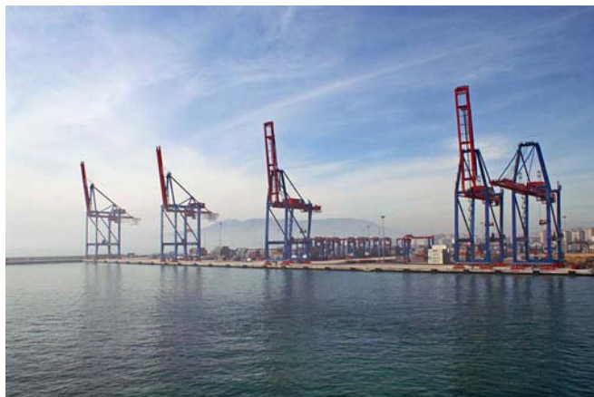
Wharf 9—Container Terminal
