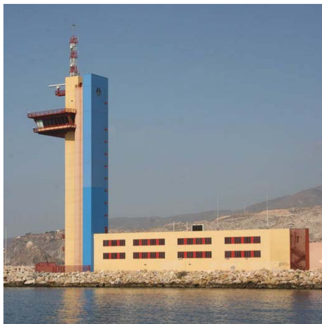
Almeria Port Control Tower
