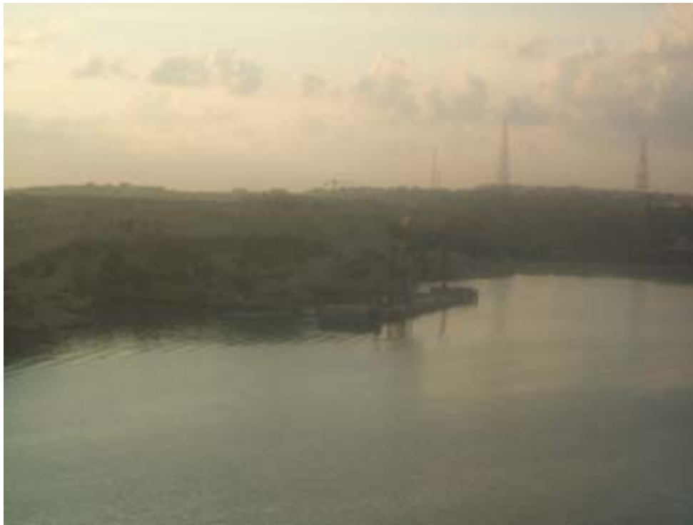
Valletta—Tank Cleaning Farm Pier
