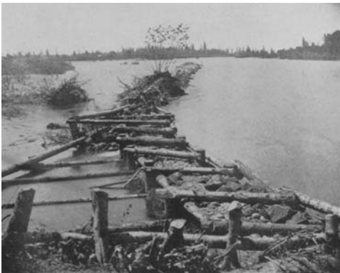
Figure 4. Skinners Bar dam, built in 1898-99 down river of Eugene. The dam served to cut off the head of a side channel and to direct water into the main channel of the Willamette (U.S. Army Corps of Engineers, 1899, as cited in Brenner 1997).
