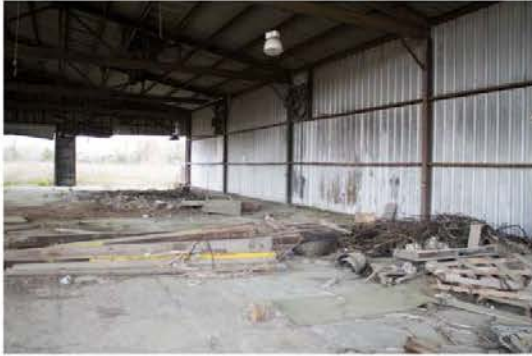
Photo 31 – Former lumber mill
