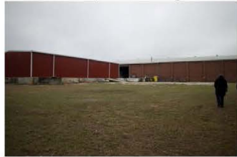
Photo 10 – Warehouse (facing south)
