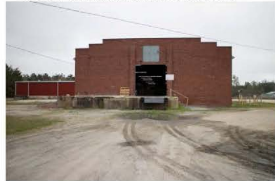
Photo 16 – Western loading dock of warehouse
