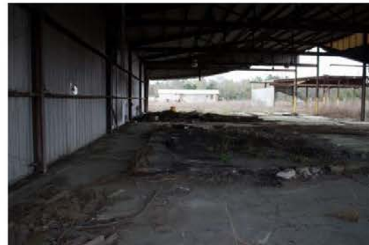
Photo 30 – Former lumber mill
