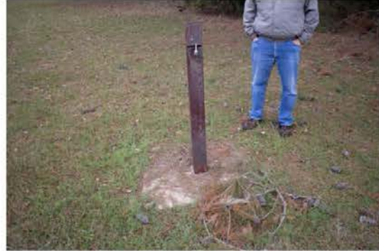
Photo 14 – MW south of recovery well and MW4
