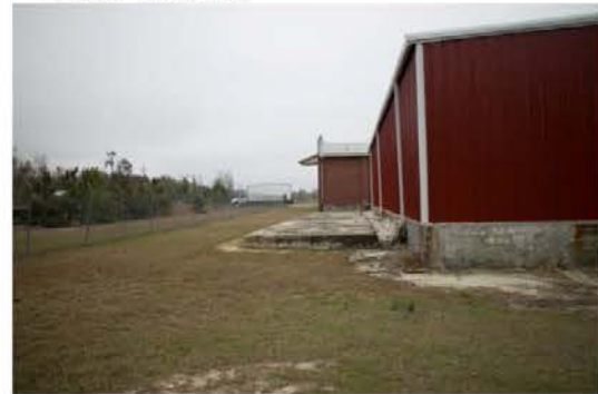
Photo 4 – Eastern side of the warehouse
