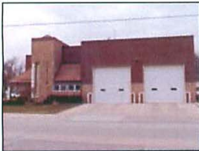
Station 4: 2622 North 15 th Street Ladder 4 Engine 6 (Reserve Engine)
