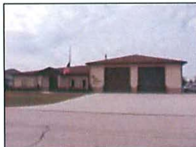
Station 5: 4504 South 18 th Street Ladder 5 Engine 7 (Reserve Engine)
