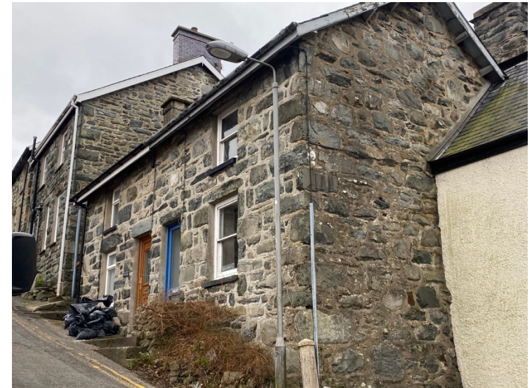
31 Buildings on Pen Dref, within the Stryd Fawr area
