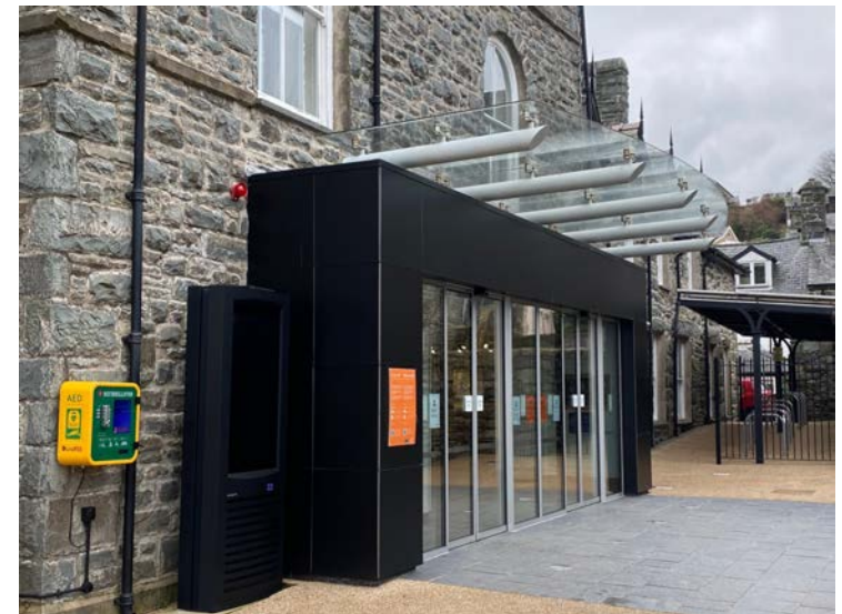
70 Modern entrance to the Castle Visitor Centre
