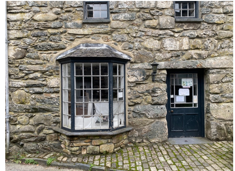
45 Stonework and window detailing at Harlech Pottery
