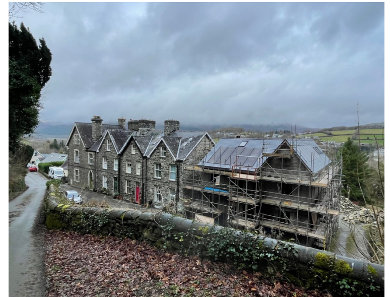
45 1-4 Bodlondeb with new house under construction adjacent. (2022).
