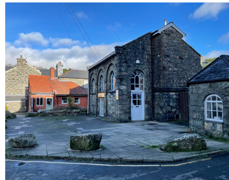
42 Former Gas Works retort house and governor house (right) (2022)
