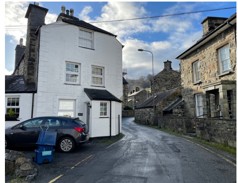
58 Poor windows and modern paint, Garn View, Heol Feurig. (2022).
