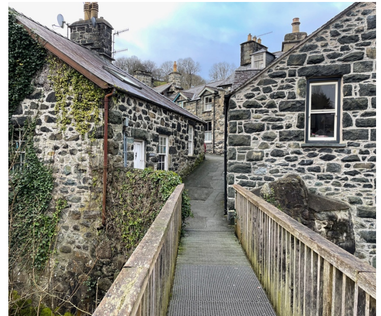
20 Across footbridge towards Maes-y-Pandy. (2022).
