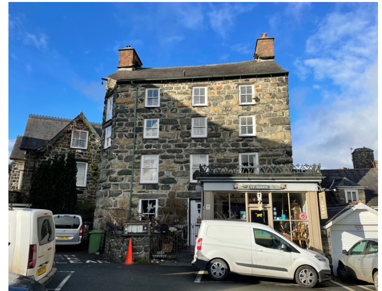
37 Ty Seren note the lifting beam. (2022).
