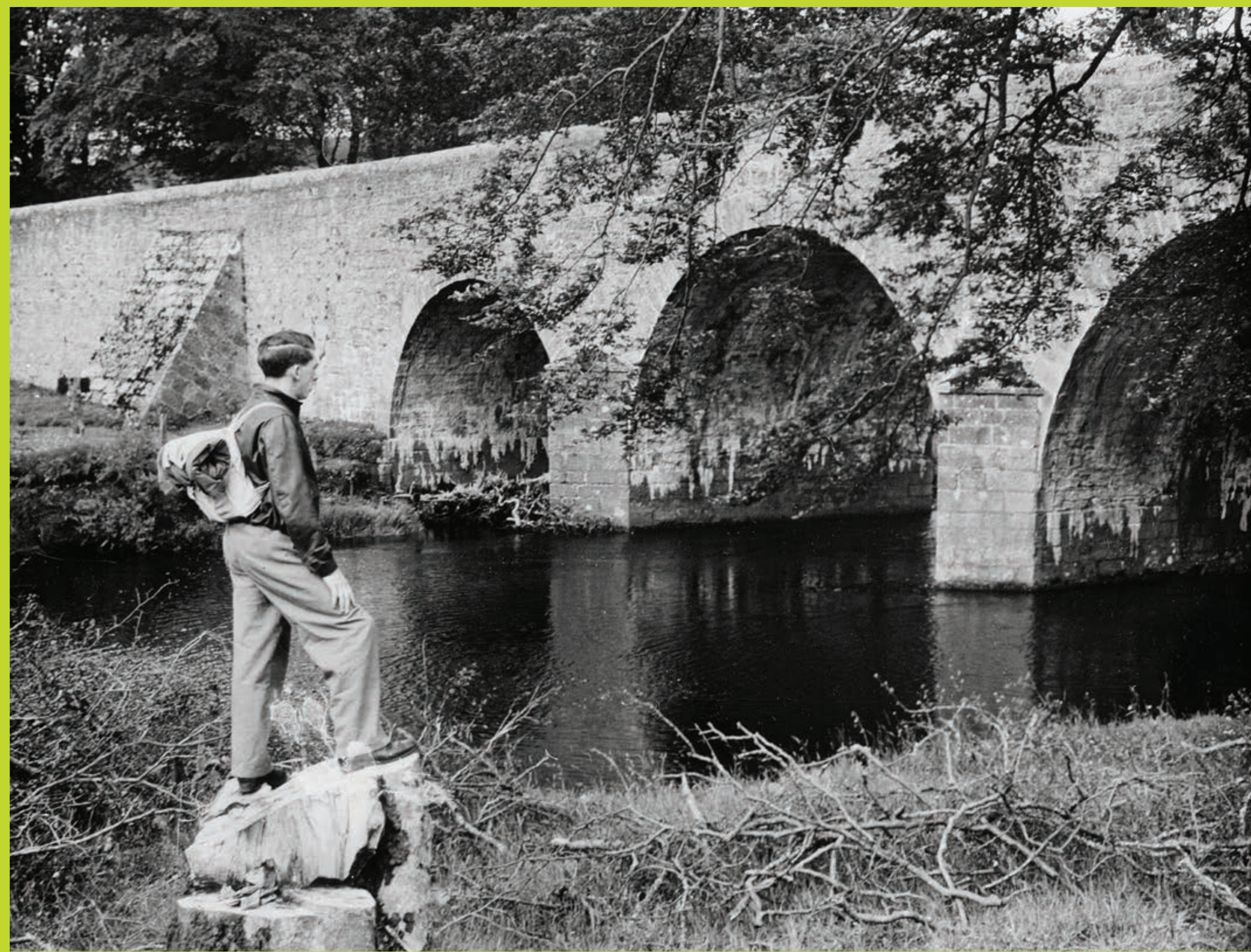
Ballyward Bridge, Kilbride, Co Wicklow
