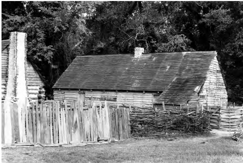
Figure 2. Three kinds of fences (pale, wattle made with twisted boughs, and scrap lumber woven and wedged between posts) at the reconstructed slave quarter at Carter's Grove. Photograph courtesy of the Colonial Williamsburg Foundation, Williamsburg, VA.
