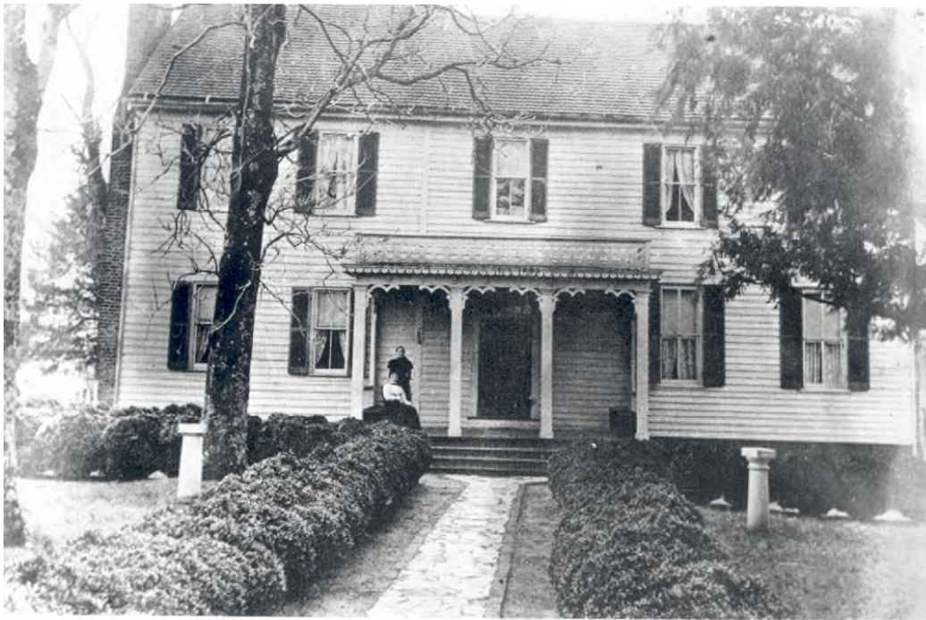
Figure 6. The Chambers House, Boydton, VA. The boxwood planted by Lucy Tucker Chambers on 7 March 1846 lines the walk leading to the front door of the house, built for Beverly Sydnor, which Edward R. Chambers (1795-1872) bought in 1843 and fitted up as the family residence. This photograph of ca. 1900 shows the façade, made symmetrical with an expansion to the east, and later two-over-two sash windows. The ladies on the porch are two daughters of Edward and Lucy Chambers.
