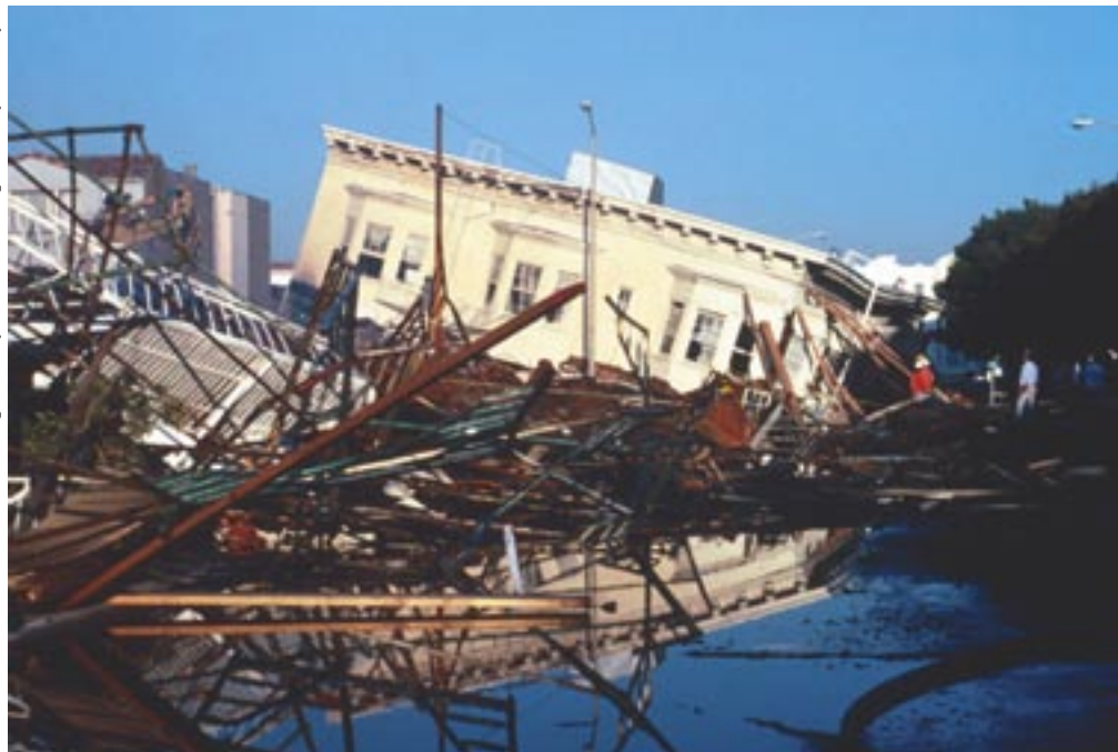
Collapsed and burned buildings shown at Beach and Divisadero streets in the Marina District, San Francisco.
