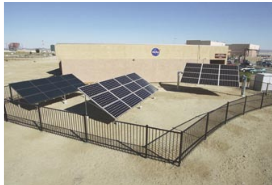
The experimental site at NASA's Dryden Research Center consists of two fixed-angle solar arrays and one single-axis Sun-tracking array. Together they produce up to 5 kilowatts of direct current power on a sunny day, which is equivalent to powering two or three average California homes. The Sun-tracking array tilts to follow the Sun using an advanced real-time tracking device rather than normal pre-programmed mechanisms.
