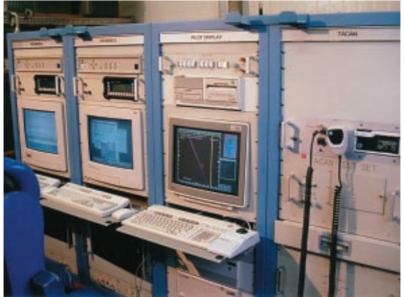
The Landing Aids Laboratory personnel at Kennedy Space Center has completed the development of a VXI bus-based miniaturized next-generation Microwave Scanning Beam Landing System (MSBLS) Flight Inspection and Certification System. The Space Shuttle uses the MSBLS to provide precision guidance during the last stages of shuttle missions prior to landing.
