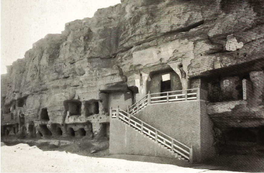
FIGURE 10.7 Main entrance to Mogao Cave 465 on top of burial Cave B42 (to the right of the lower steps of the staircase) and Cave B43 (to the left of the lower steps of the staircase)
