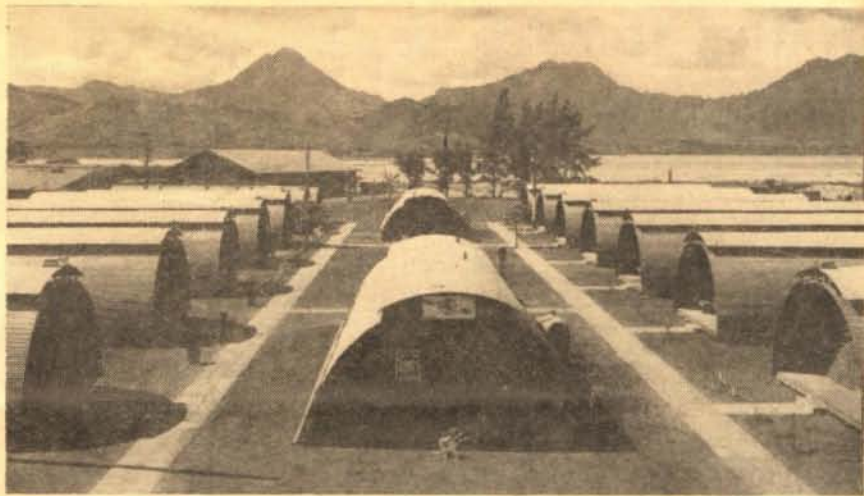
Shown here during one of its quieter hours is the CBMU enlisted men's quarters. The 16 huts are tropical-type units, and recently were constructed by the CBMU for their own use during their stay here.
