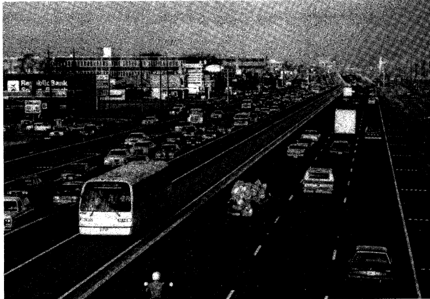
Busways in Houston are constructed within the existing median of the freeway and protected by concrete barriers (above). Support facilities include park-and-ride lots (below).
