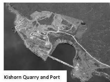
Kishorn Quarry and Port
