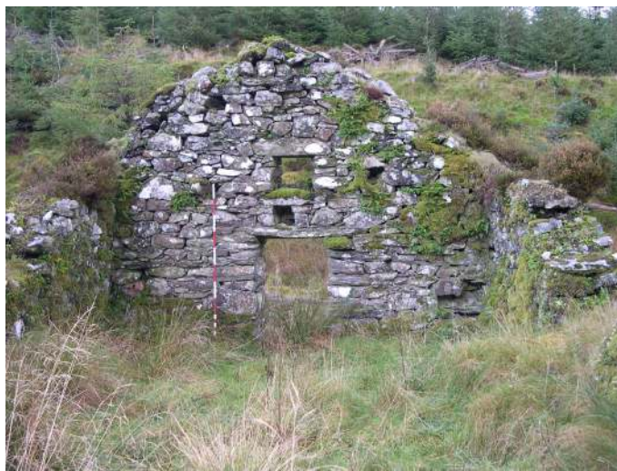
Site 352 Craigmurraill, Structure 2 internal gable end
