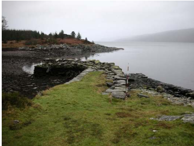
386 West Otter Ferry pier and slipway
