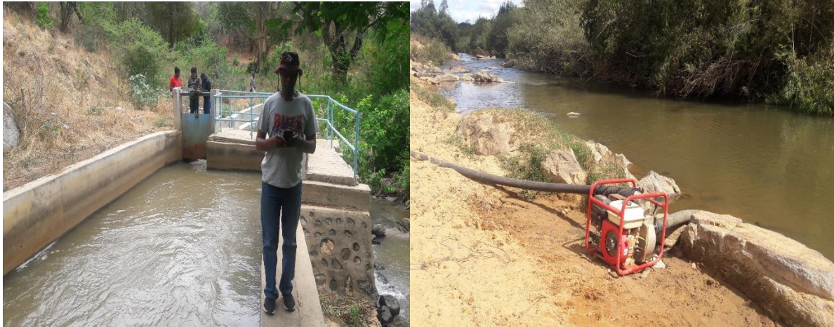
Photo 5: Water pumping and Intake for irrigation along Little Ruaha River in Iringa district. Source: IRA and SUA survey Team, 2019
