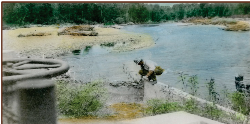
A tribal diversion on the Pine River circa 1927. This same diversion structure is still in use, despite its antiquated condition.
