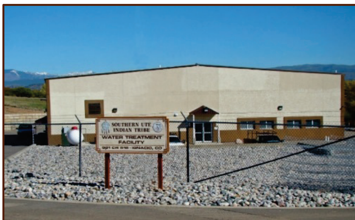
The treatment plant for the Ute municipal system that serves the Southern Ute Indian Tribe campus, the Town of Ignacio, and close to 350 residences via 19 miles of pipeline.
