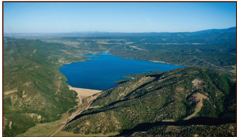
The A-LP Project's Ridges Basin Dam and Reservoir, Lake Nighthorse, near Durango, Colorado.
