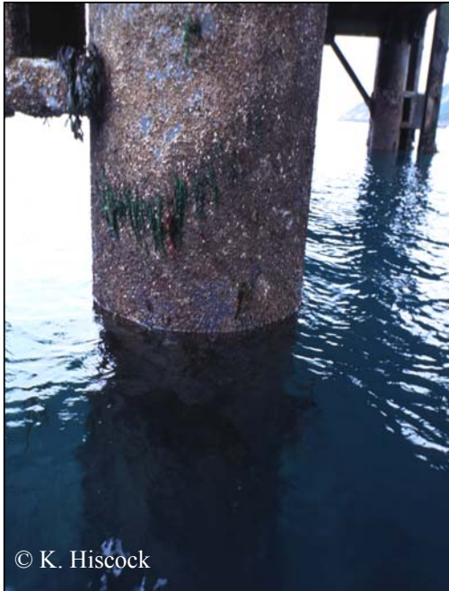
Plate 9. Intertidal communities dominated by barnacles with green foliose algae. Similar to the community likely to develop on offshore wind farm structures. Jetty pile diameter approx 1.5m.
