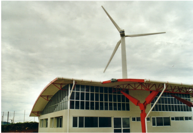
Fig. 4 Wind power plant control building at Tejona, near wind turbine position #30.
