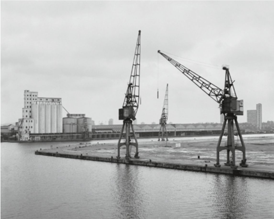
Mike Seaborne, Derelict Millwall Docks looking south west towards the McDougall's grain silos, 1982
