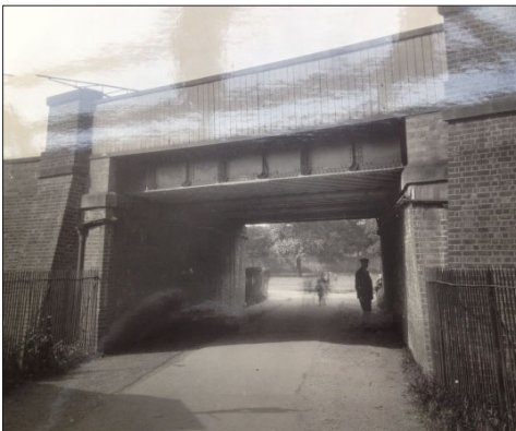
Railway bridge for the West End and Crystal Palace line (1930). Reproduced courtesy of London Metropolitan Archives, (City of London).
