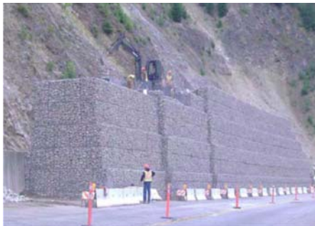
Gabbion basket/wire mesh wall.
