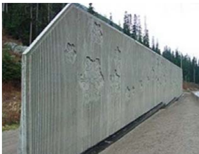
Reinforced concrete wall
