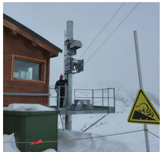
Figure 29. CATEX aerial tramway base station in Saint Francois Longchamp ski resort, France. A. Jones photo.
