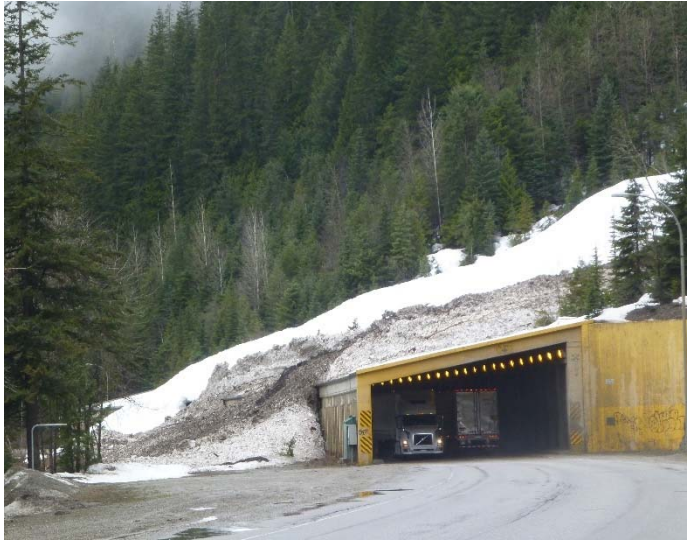
Figure 13. Two-lane concrete Lanark snow shed in Rogers Pass, British Columbia. A. Jones photo.
