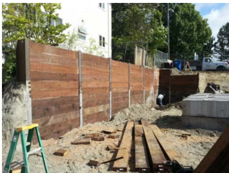
Soldier Pile wall (H-Piles and timbers)
