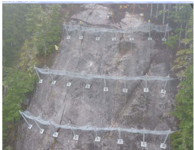
Figure 12. An example snow net installation at 35 Mile Bluffs, BC, Canada. Photo: A. Jones.
