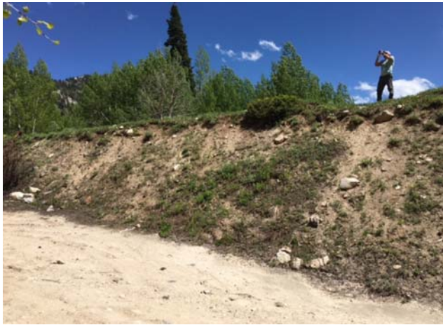
Figure 15. Earthfill berm in Emma 5 (Culps West) to protect residence.
