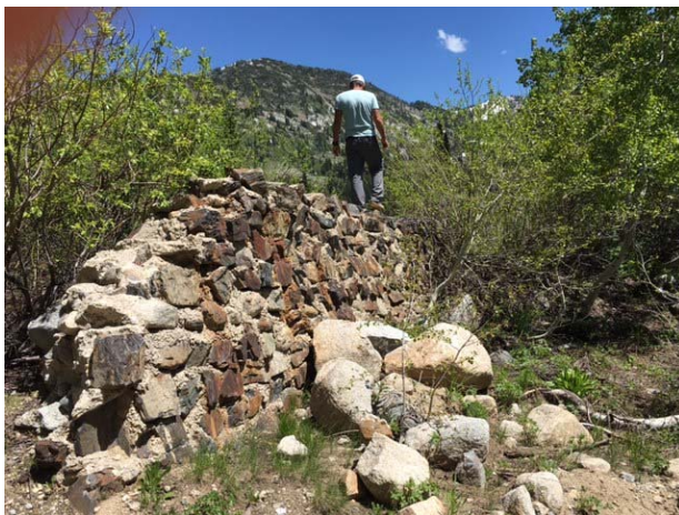
Figure 17. Stacked rock diversion wall in Emma 1 path, near TOA water reservoir.
