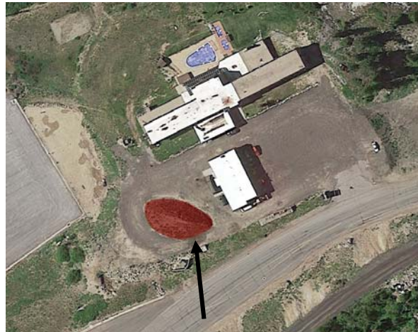
Figure 16. Earthfill berm (highlighted in red, with arrow) in front of the Peruvian Lodge.
