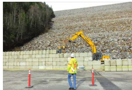
Concrete block wall (Lock-blocks)
