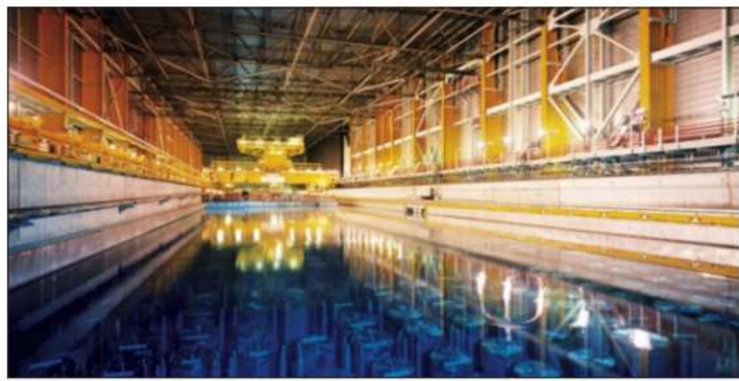
Figure 1: Spent fuel storage pond at Sellafield. Taken from [1].
