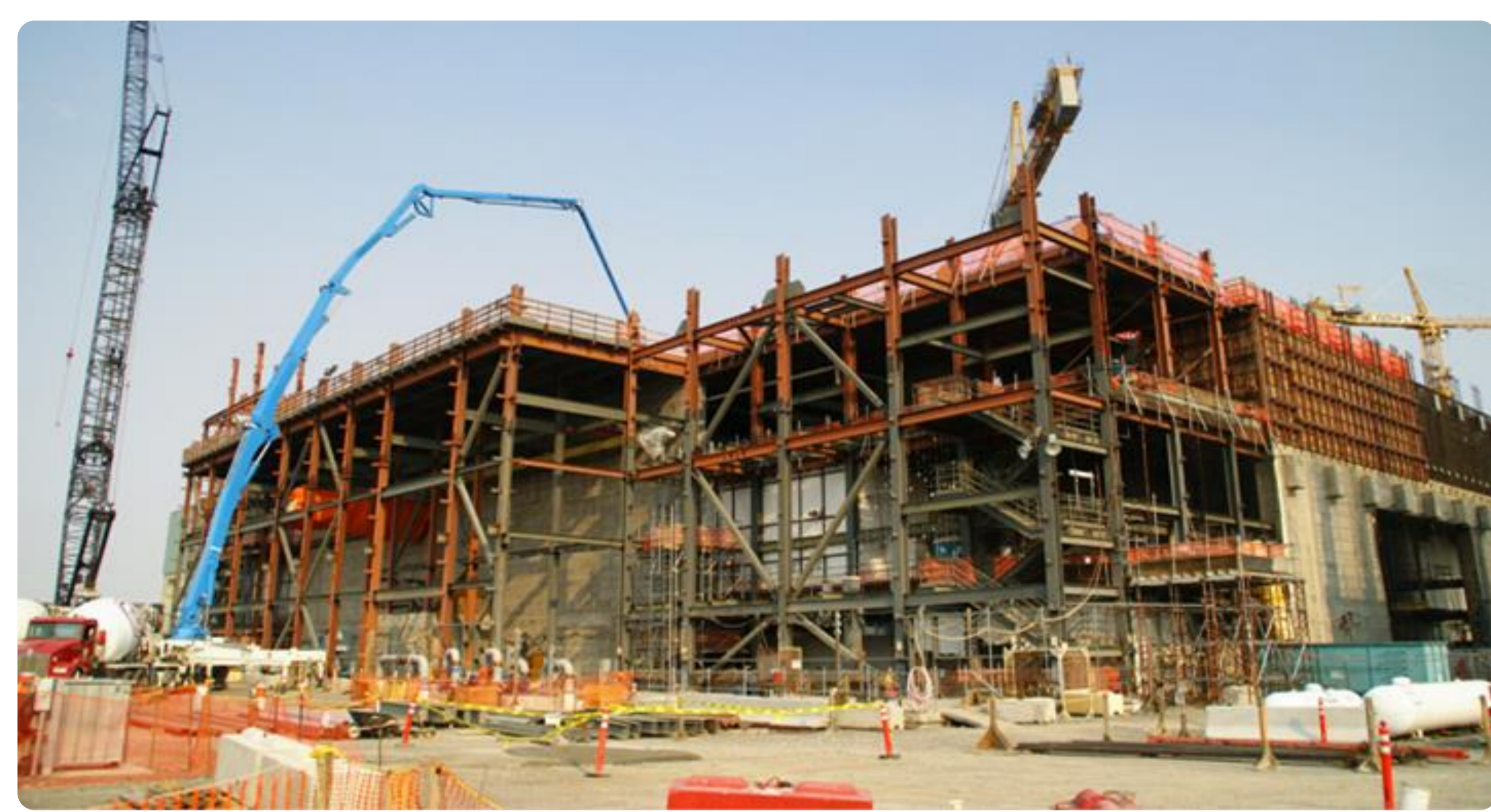
Fig 1. The Hanford Waste Vitrification Plant currently under construction 1 .
