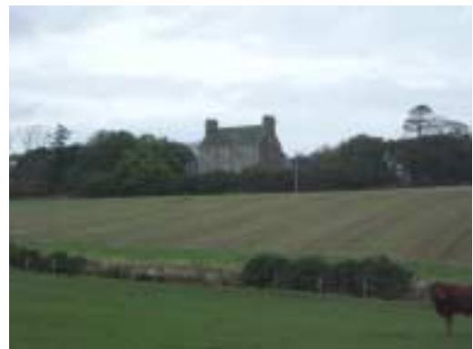
Orrock House (A-Listed)
