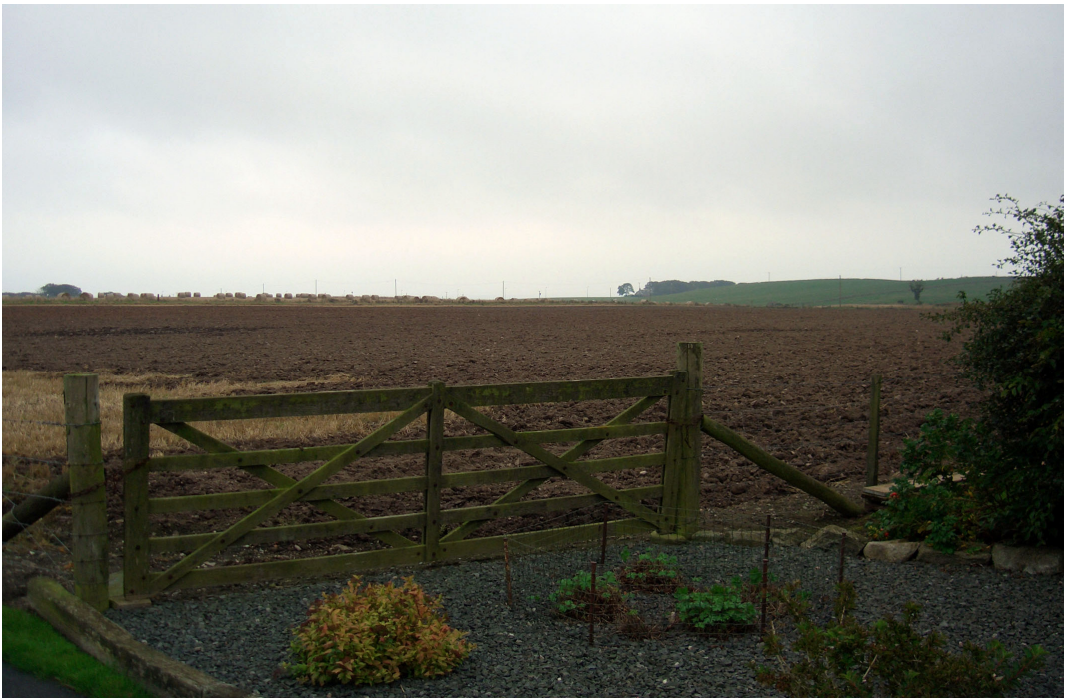
Figure 11.18. View from Kirkhill. New road on embankment (tapering down from right to left) across the whole of the view (towards the rear of the ploughed field), gives rise to major adverse visual effects in the short term, reducing to moderate as mitigation matures
