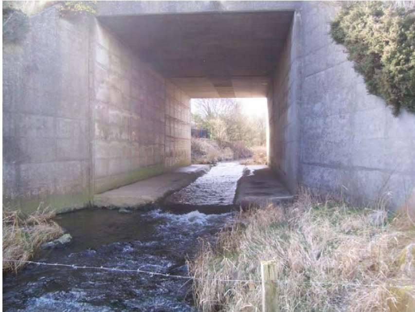
Photograph 5 – Current A90 culvert with low flow channel (looking west)
