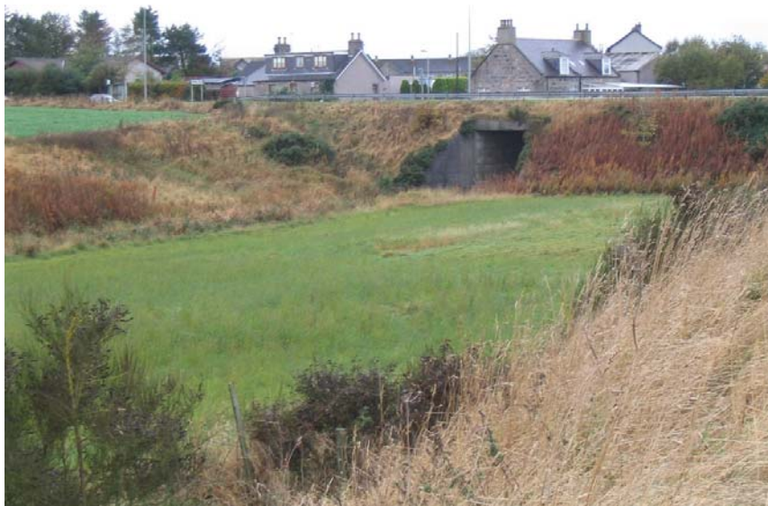
Photograph 4 – Embankment and culvert on current A90 embankment (looking west)
