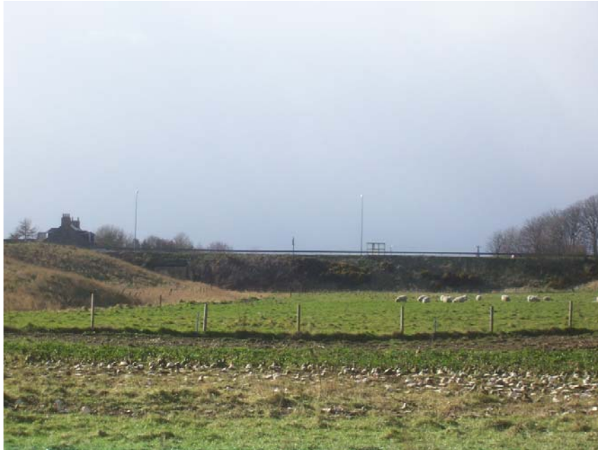
Photograph 1 – Current A90 embankment (looking west)
