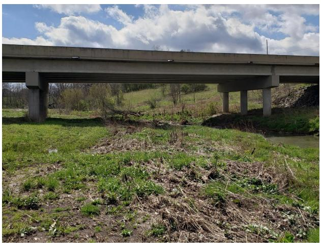
Image 5: Looking south along tributary to Hardins Creek under KY 2154. Notice the vegetation bent by water flowing beyond its banks.
