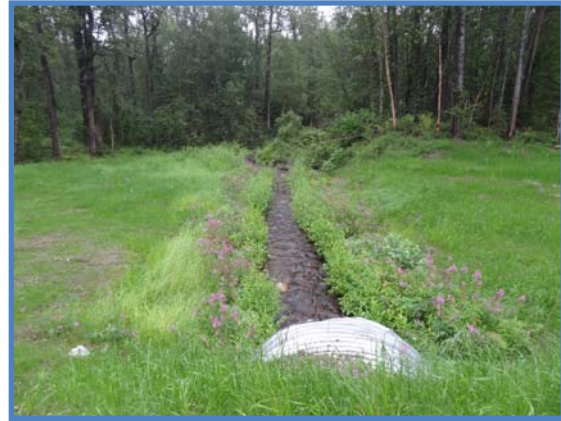
Indian Creek culvert replacement site after revegetation work, August 2013.
