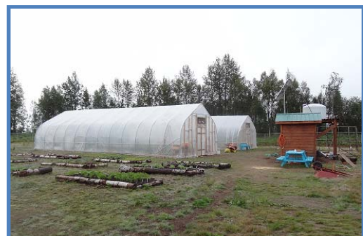
Newly constructed high tunnels in Tyonek community garden, June 2013.
