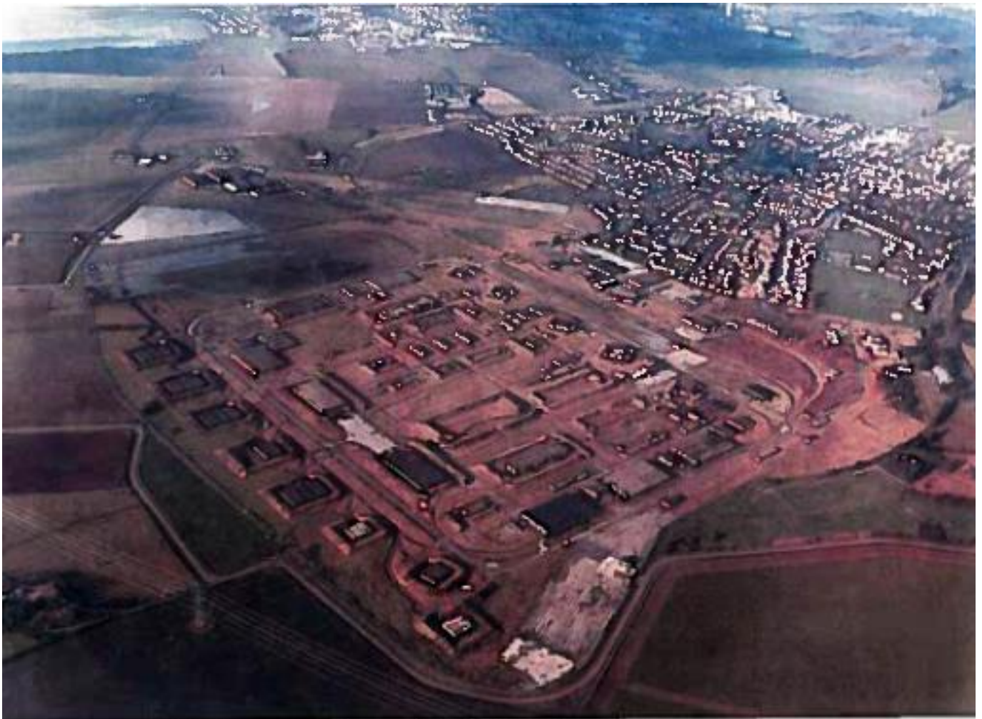
An aerial view of the Depot site in 1989, just before demolition began.
