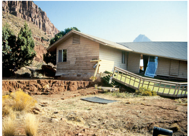
A landslide caused by the 1992 St. George earthquake destroyed this house in Springdale.
