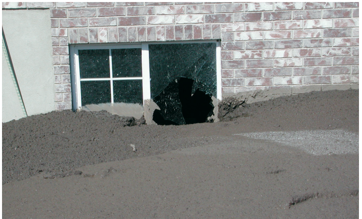
The debris-flow impact broke through the basement window of this house on Apple View Street in Santaquin.
