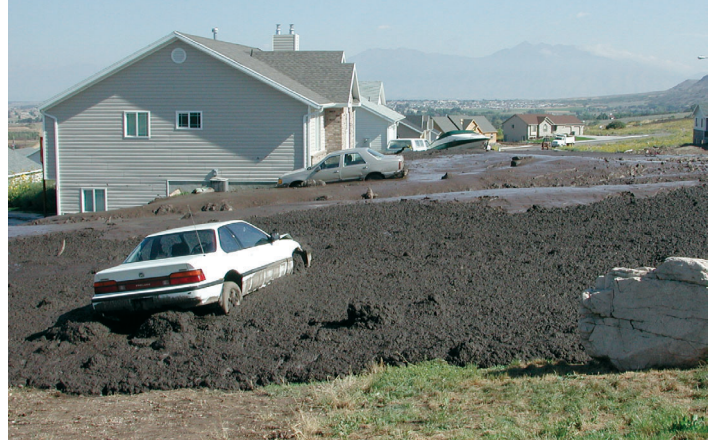
Sediment deposited at the intersection of Lambert Avenue and Apple View Street in Santaquin. The debris flow moved cars and filled basements with sediment.
