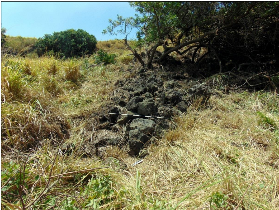
Figure 33. Site 29231 Feature C, eastern wall of the lower level area, view to the southeast.
