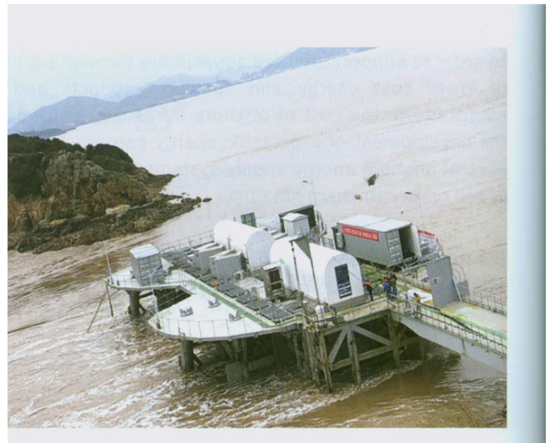
LHD Tidal Current Energy Demonstration #1 Platform – China
